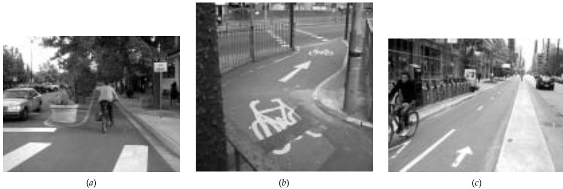
Separated Bicycle Facilities (SBF's) come in all shapes and sizes: (a) contra flow lane in downtown Boulder, CO; (b) specialized treatment at an intersection near Swiss Cottage, London; and (c) a downtown corridor in Montreal. While increased safety is a primary justification for these treatments, the bulk of the available research is unable to confirm reliably this. Nevertheless, they appear to increase perceived safety among select groups such as the elderly, children, and inexperienced cyclists.
